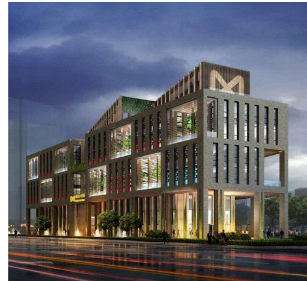
BREEAM Outstanding for Living Lattice exhibition centre China
