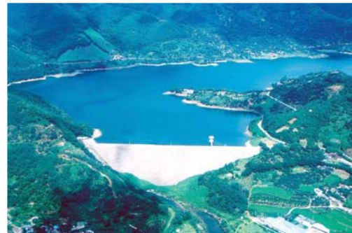
Gwangyang small-hydro power plant in Jeon-nam province
