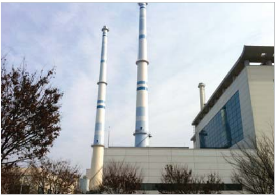
Biomass cogeneration in Korea District Heat Corporation
