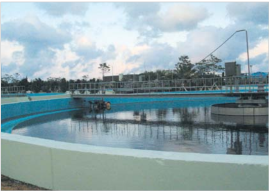
Jeju Bio cogeneration plant
