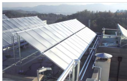
Solar water heating system in Daedeok
