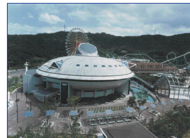
Solar Energy Park in Daejeon
