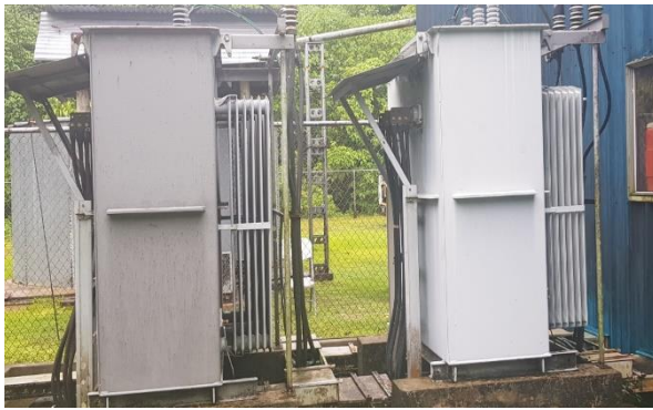
Figure 15. Main Transformer in Diesel Power Plant (1,000kW x 2)
