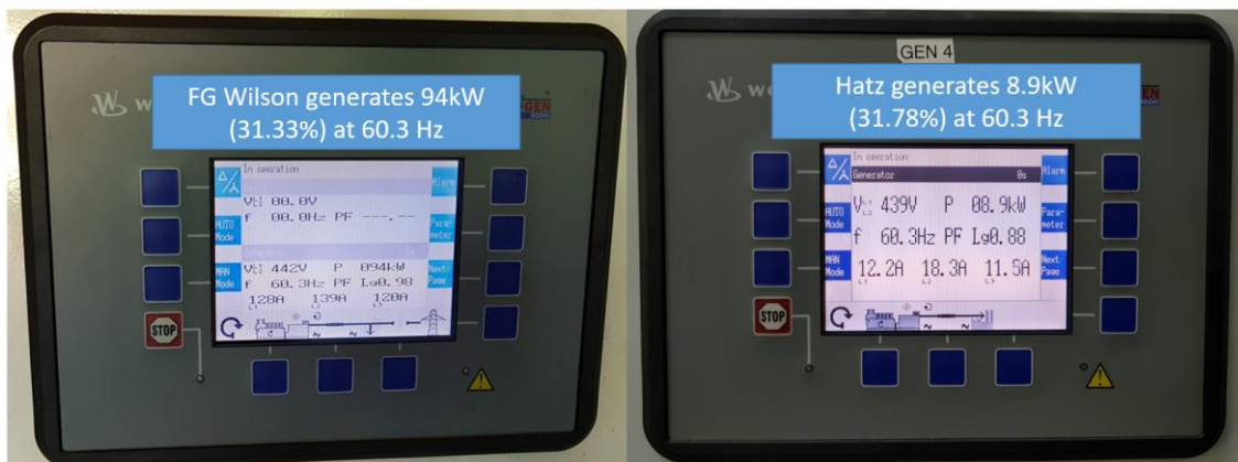
Figure 21. FG Wilson and HATZ generators share the load corresponding to their nominal power at 60.3 Hz.
