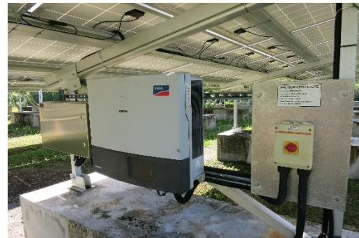
Figure 17. SMA Inverter in PV Plant.
